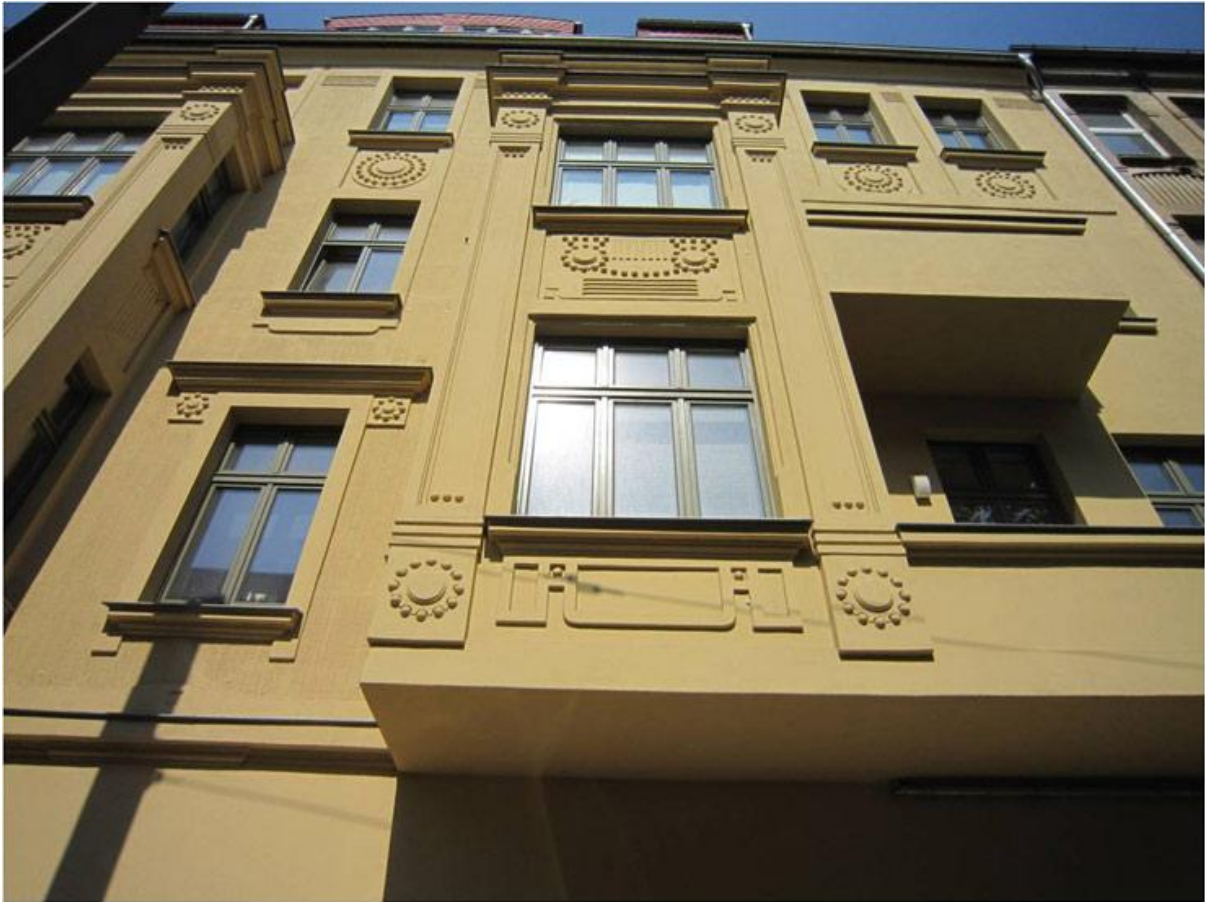
Property post renovation
